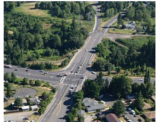
Long-awaited interchange to replace St. Johns Boulevard-Highway 500 intersection, above, to get underway in 2010.
